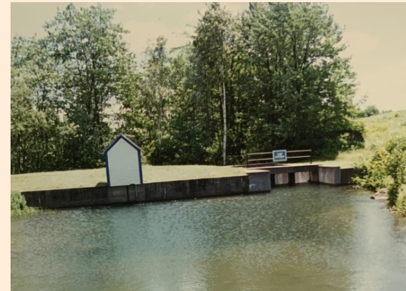
1996 views of upstream face with gate house and downstream face of stop log bays (NHDES).
