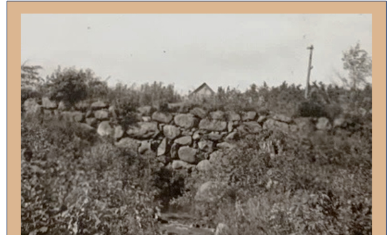
Early twentieth century view of downstream face shows underlying stone dam before it was rebuilt by the electric company (NHDES files).
