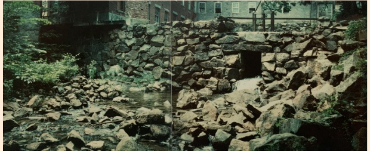
1982 downstream face of lower dam with outlet gate open (NHDES).
