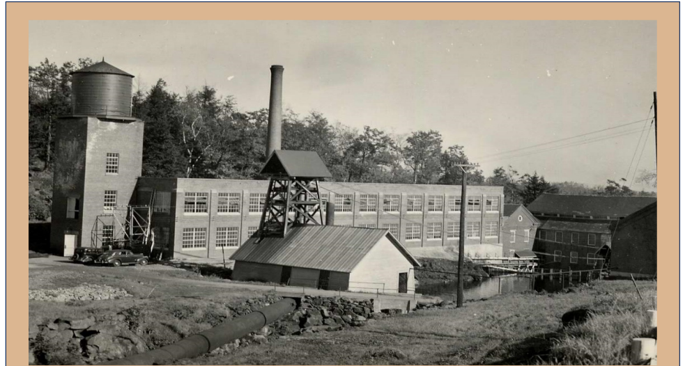
Looking downstream in the 1930s, showing penstock pipe to the powerhouse. Tower on top is the upper end of the rope drive system transferring power to the Cheshire Mills below. The rope drive was used until the plant was fully electric in 1948. The wheelhouse was taken down afterwards (Historic Harrisville, Inc. Archives).
