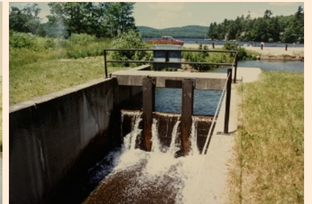
1996 views of upstream face with gate house and downstream face of stop log bays (NHDES).
