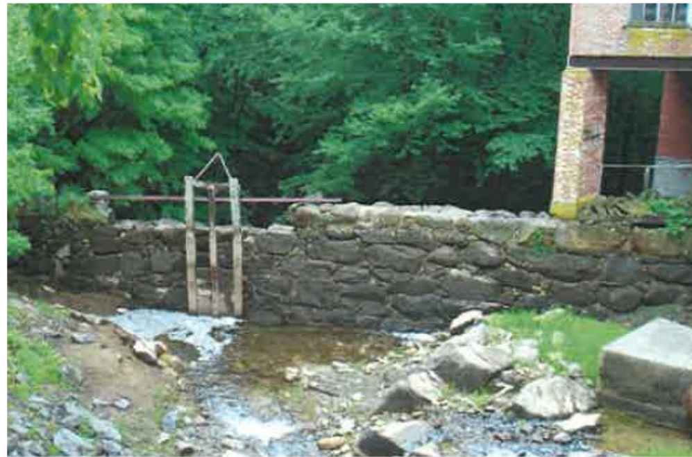
Upstream face of Lower Dam in low water (NHDES).
