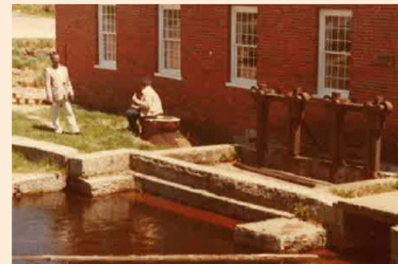
Harris Mill and dam in 1978 shows the four rack and pinion gate mechanisms (NHDES).
