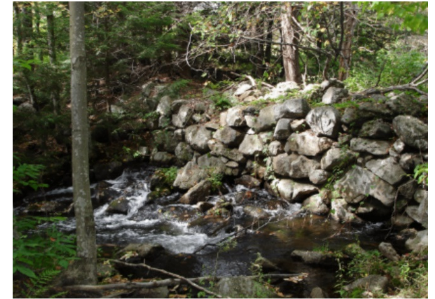
Mosquitobush mill foundation walls (Historic Harrisville, Inc.).
