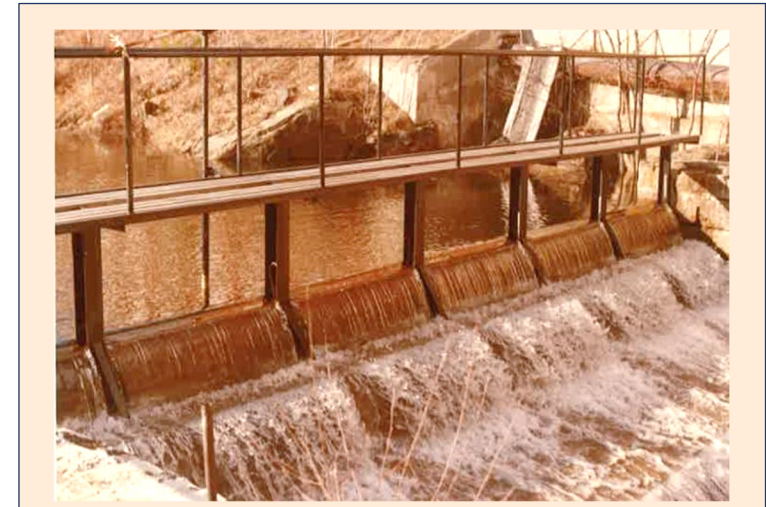
1979 photo of spillway, downstream face (NHDES).
