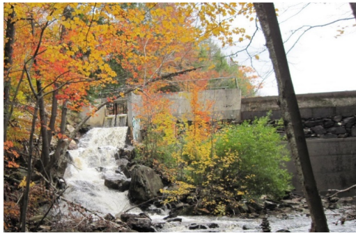
Downstream face with sluiceway open, 2010 (NHDES).
