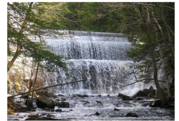
Howe Reservoir Dam downstream face of spillway in high water (NHDES).
