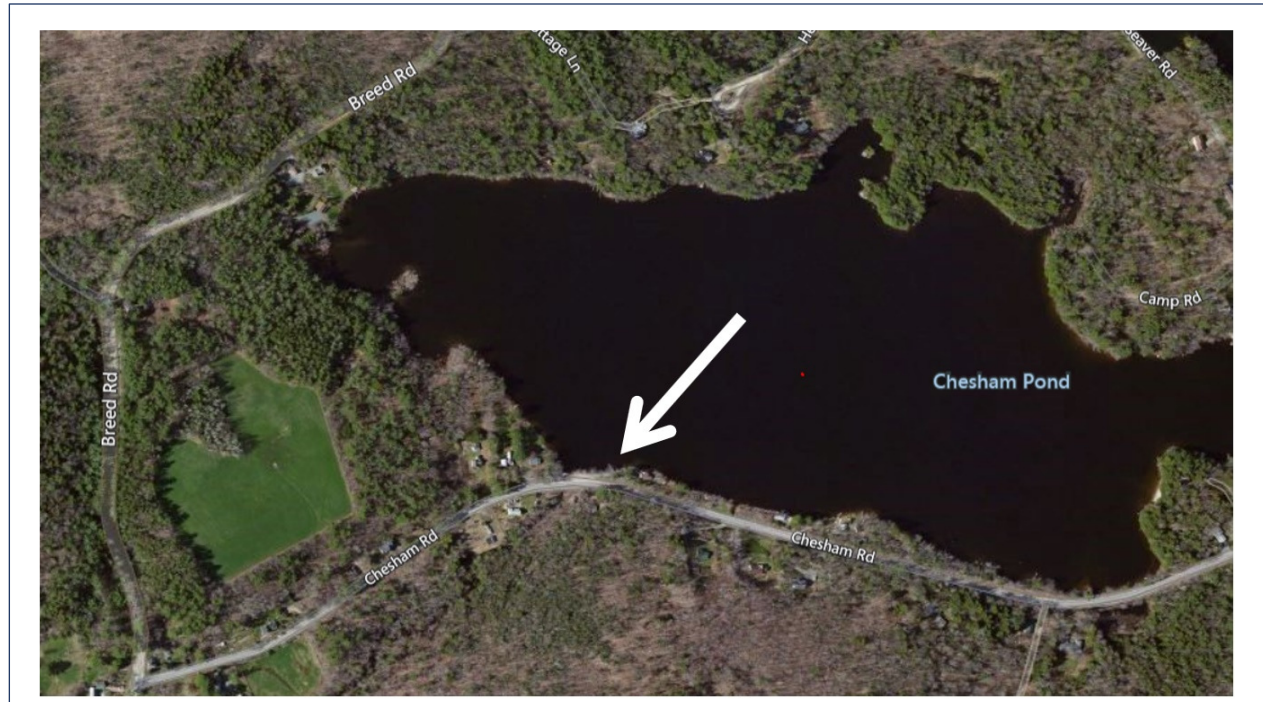
Chesham Pond Dam.
