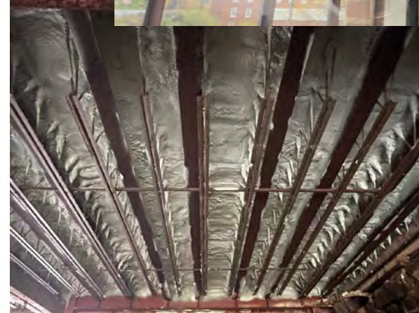
Closed cell foam insulation was added beneath the exposed floor of Mill No. 5, built by Filtrine in 1985. The space above, which was formerly storage, now houses Harrisville Designs' shipping department .
