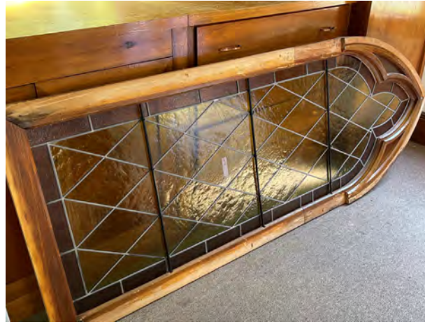
A restored stained glass window awaiting reinstallation.
