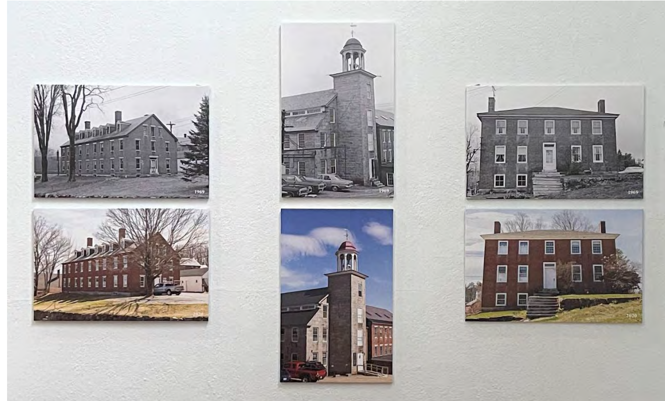
A photo exhibit of Harrisville buildings in 1968 and 2020 illustrates the amazing historic preservation work that has occurred in Harrisville more than 50 years. The cars and trees have changed, but the buildings remain the same!
