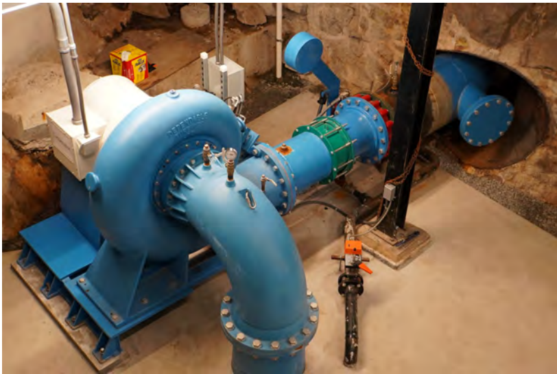
Because of the unusually wet summer, the turbine was operating so visitors could see and hear it using water to generate electricity for the Cheshire Mills Complex.
