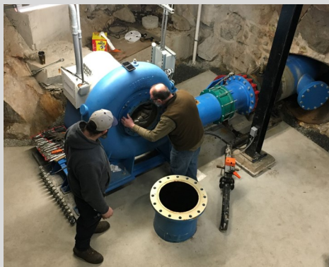
Cleaning the turbine to remove frozen leaves and twigs to restore efficiency.
